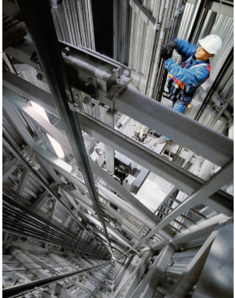
▲ Kone's high-rise test laboratory in Tytyri, Finland
